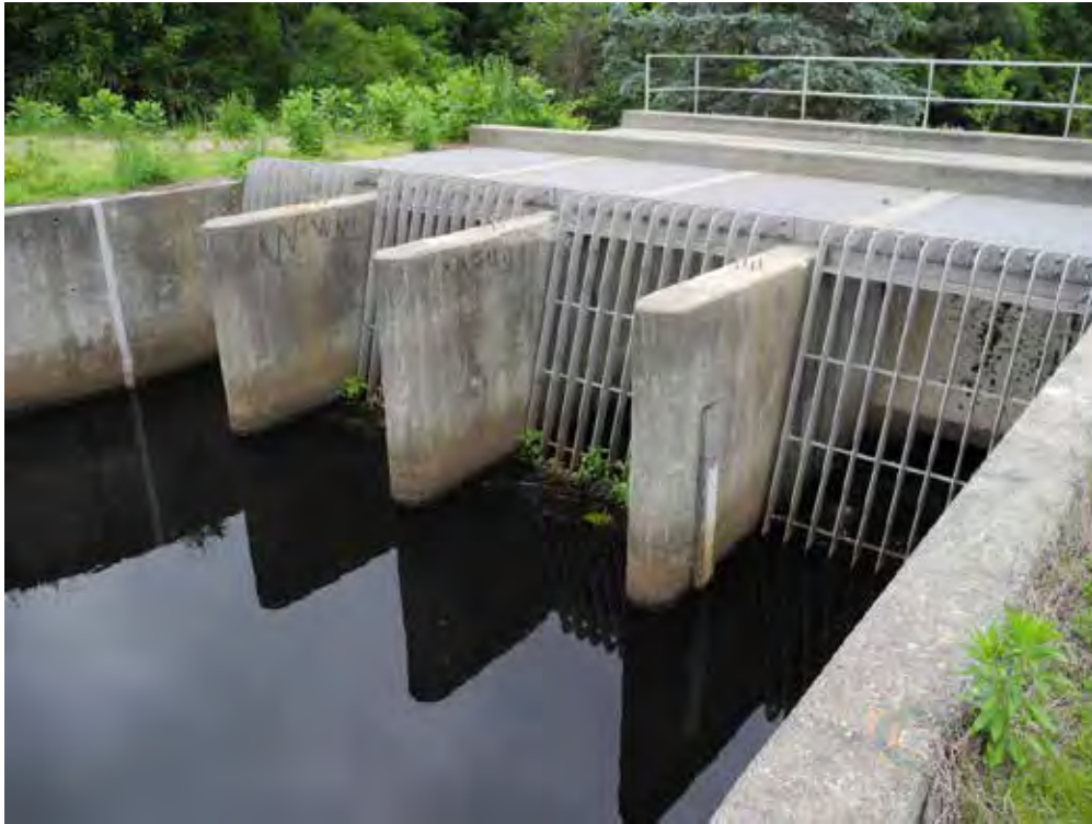
Siphon spillway inlets (GSE, 6/11/14)
