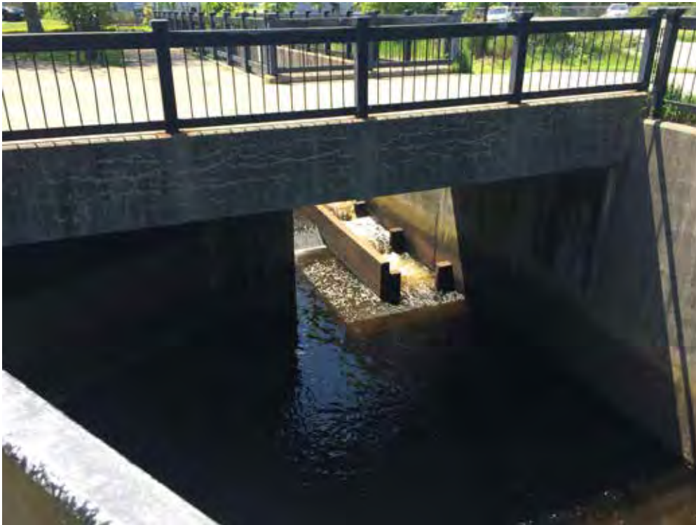
Looking upstream; note elevated concrete deck above existing swing gate (GSE, 5/25/14)
