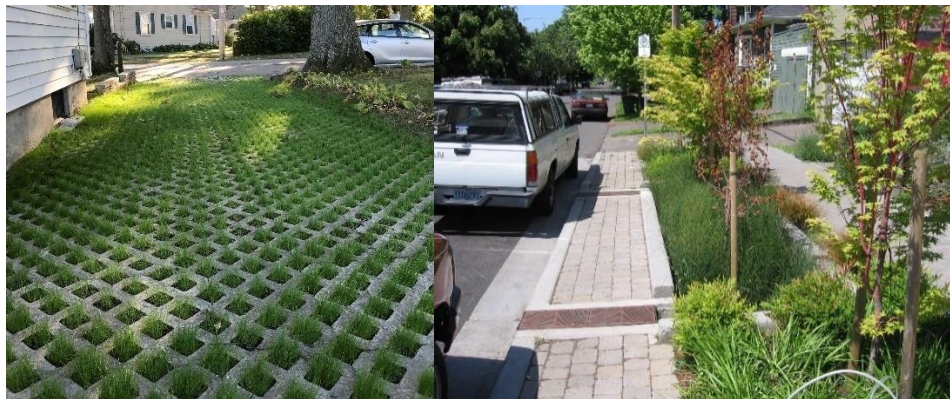
Examples of green infrastructure/LID to manage runoff and remove pollutants in stormwater.
