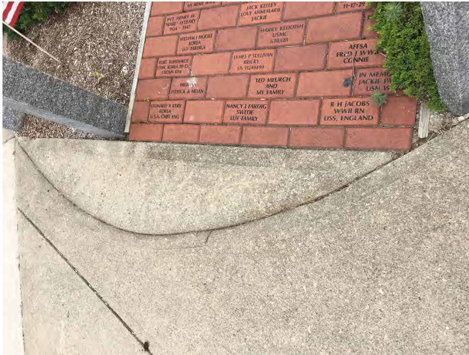
This portion of sidewalk is poorly graded to access memorial brick walkway
