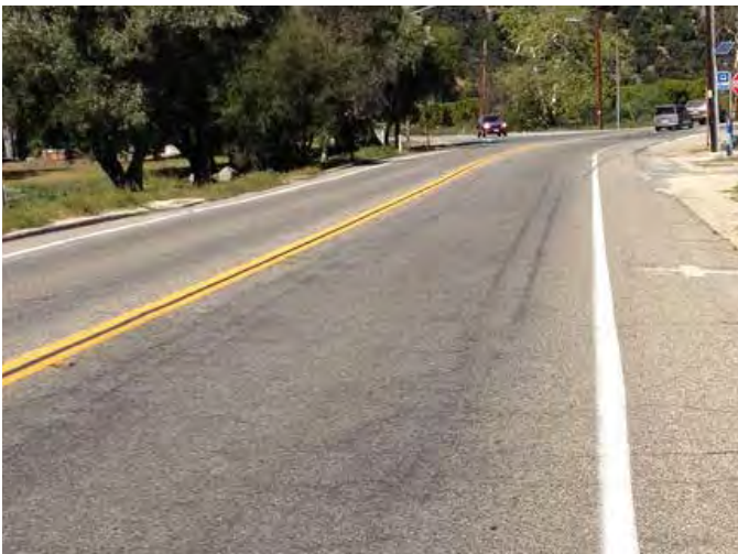
Fog lines delineate the vehicular driving zone on wide roadways.
