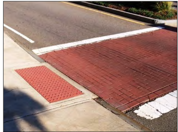
Figure 2-5: High-contrast grade changes, a detectable warning strip and ADA-compliant curb ramp. Photo by Nicholas Bulens
