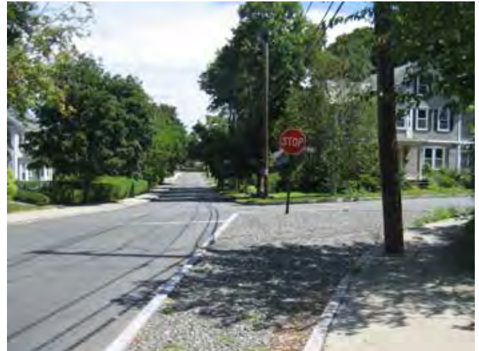
(A) Gravel-filled curb extension
