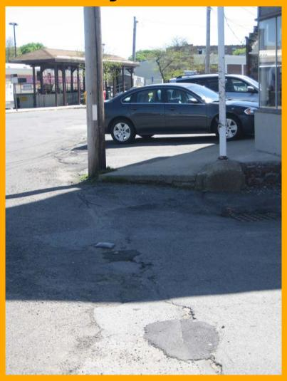
Needs attention – no curb ramp, wide driveway, narrow sidewalk, broken asphalt
