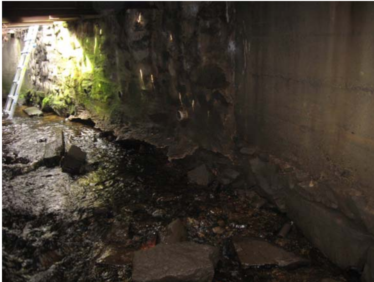
Smelt Brook 5 - view showing undermining along north culvert stone wall.
