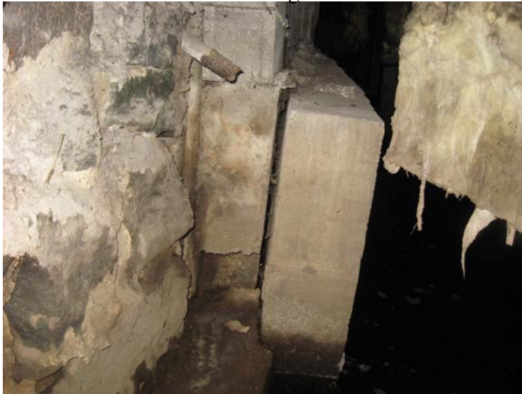
Smelt Brook 14 - view looking toward Commercial Street showing movement at culvert walls.
