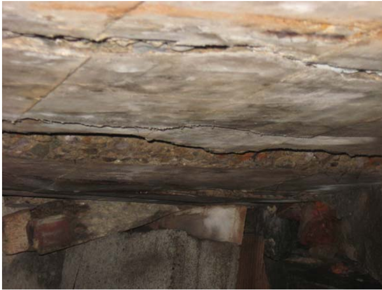
Smelt Brook 31 - view of reinforced concrete slab at Commercial Street sidewalk showing significant deterioration.
