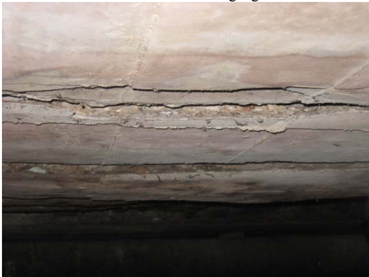
Smelt Brook 27 - view of reinforced concrete slab at Commercial Street sidewalk showing significant cracks.
