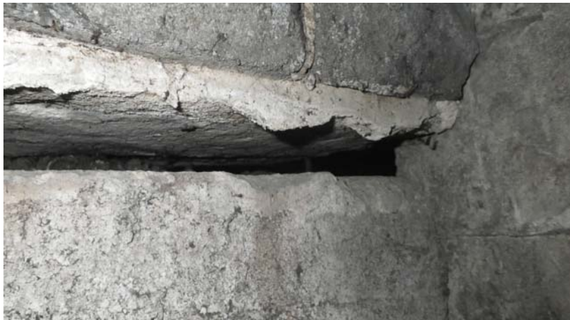
Morante Insurance/Barber Shop Basement M6 - view showing significant settlement of basement wall and concrete cap.
