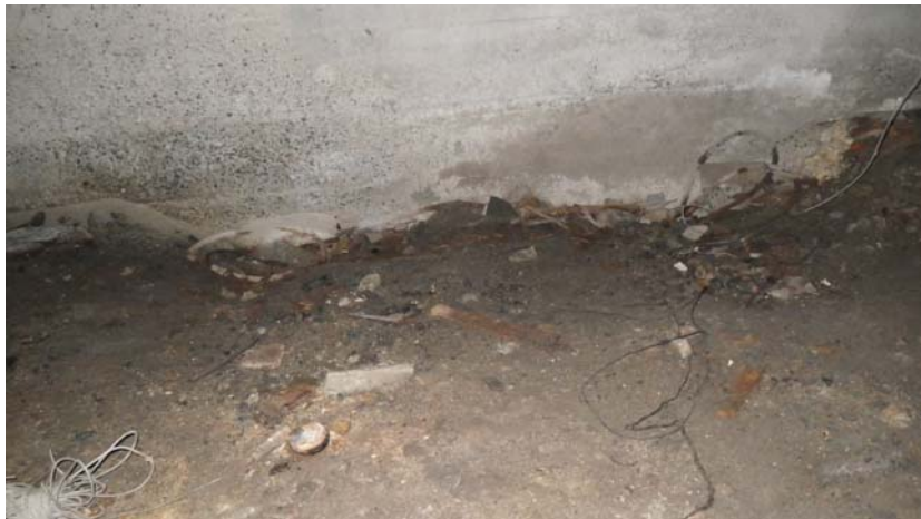
Morante Insurance/Barber Shop Basement M11 - view shows settlement of soil in basement.
