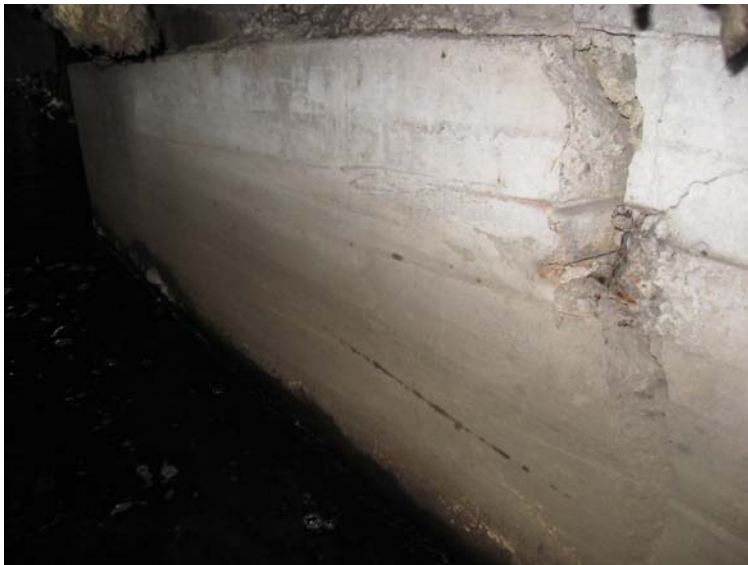
Smelt Brook 17 - view looking away from Commercial Street showing cracked and settled wall.
