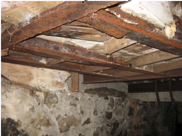
Smelt Brook 9 - view of deteriorated steel floor framing above culvert.
