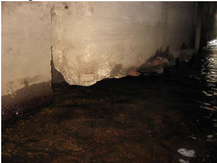
Smelt Brook 18 - view looking away from Commercial Street at undermined wall section below.
