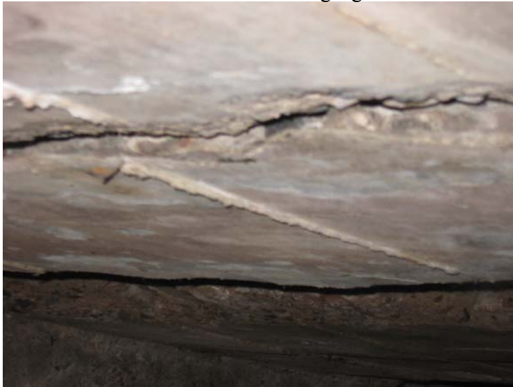
Smelt Brook 29 - view of reinforced concrete slab at Commercial Street sidewalk showing significant cracks.
