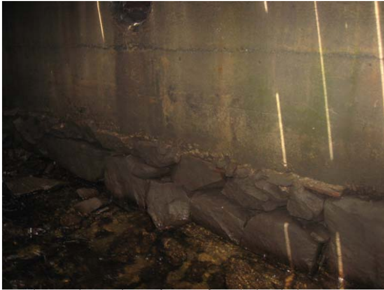
Smelt Brook 4 - view of stone foundation below concrete wall along north side of culvert.
