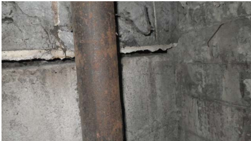
Morante Insurance/Barber Shop Basement M8 - another view showing settlement.
