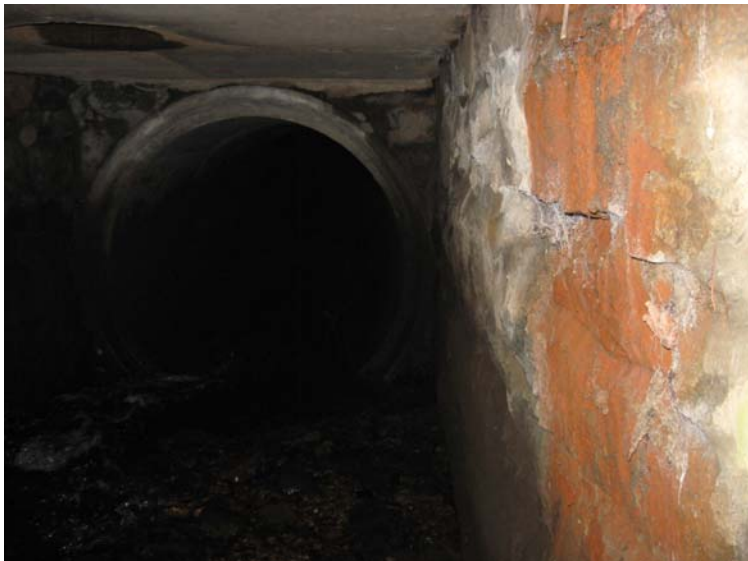
Smelt Brook 3 - looking east at 72 inch pipe beneath concrete slab.
