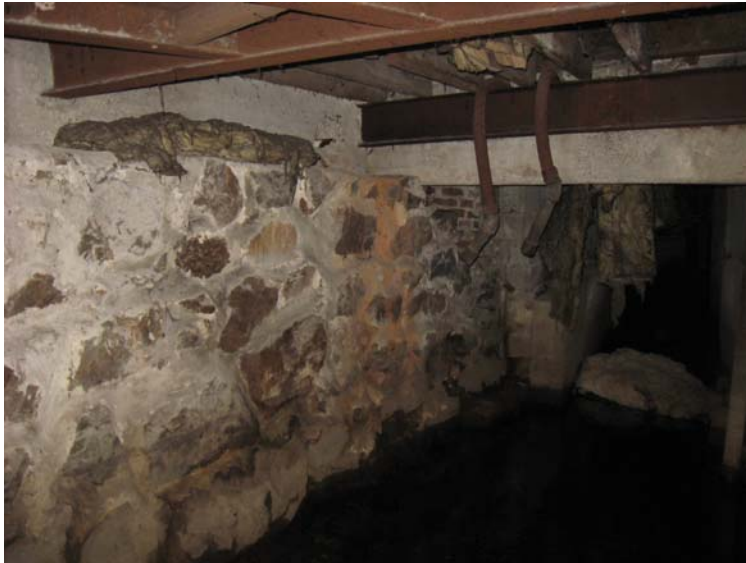
Smelt Brook 11 - view looking at additional steel floor framing.
