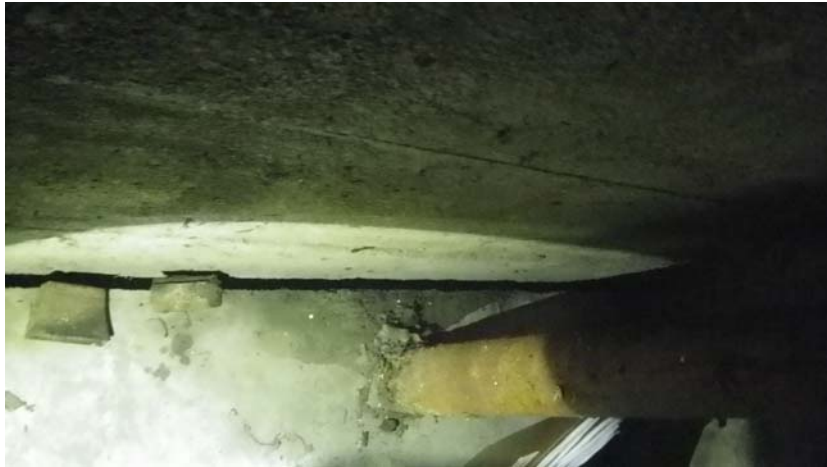
Morante Insurance/Barber Shop Basement M7 - view along culvert wall showing separation of slab and wall.
