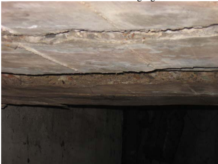
Smelt Brook 30 - view of reinforced concrete slab at Commercial Street sidewalk showing significant cracks.
