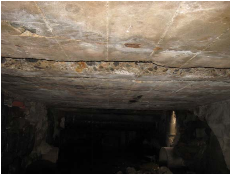
Smelt Brook 26 - view of reinforced concrete slab at Commercial Street sidewalk showing significant deterioration.
