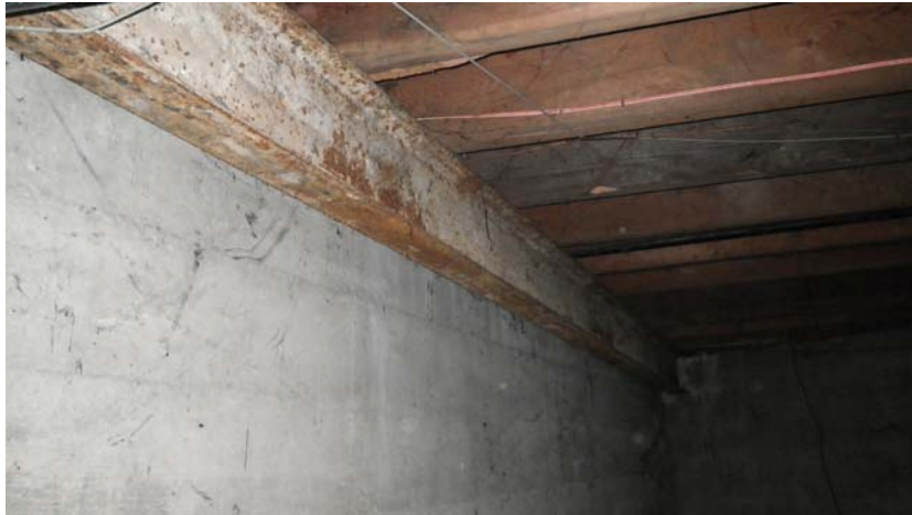
Morante Insurance/Barber Shop Basement M10 - view showing steel beam framing of floor above.
