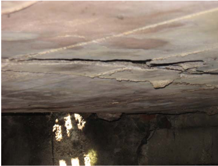
Smelt Brook 28 - view of reinforced concrete slab at Commercial Street sidewalk showing significant cracks.
