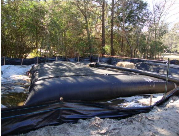
Geotubes used to dewater hydraulically dredged material
