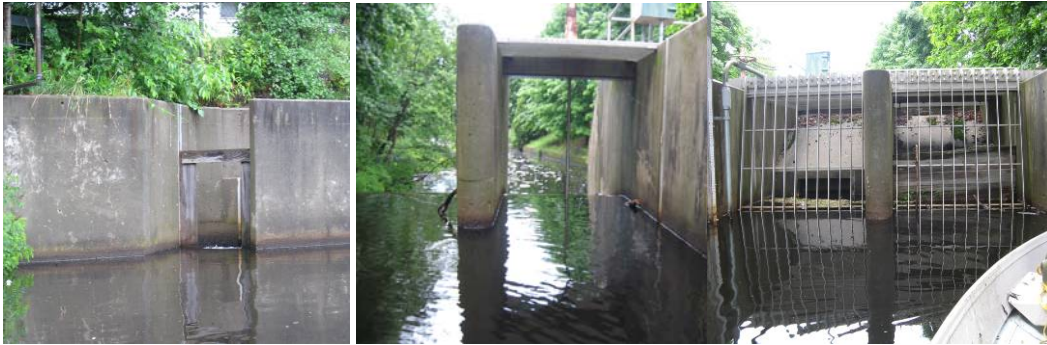
Outlet structures at Whitman's Pond include the fishway (left), main spillway (center), and flow diversion gates (right).
