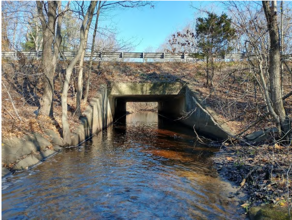
Figure 8: Upstream face of Route 3 (Pilgrims Highway) northbound crossing
