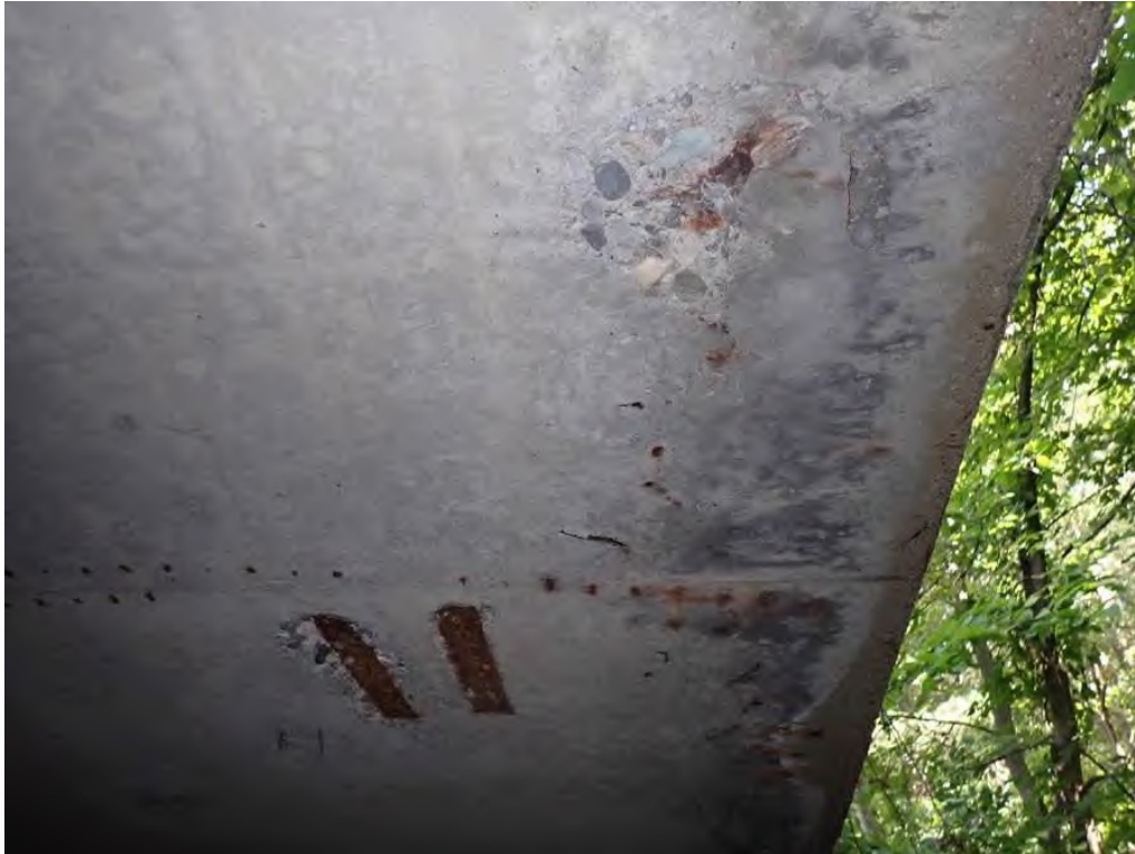
Photo 5: East end of roof, two 2" x 10" exposed metal, one with delamination and minor spall just south of exposed metal at midspan
