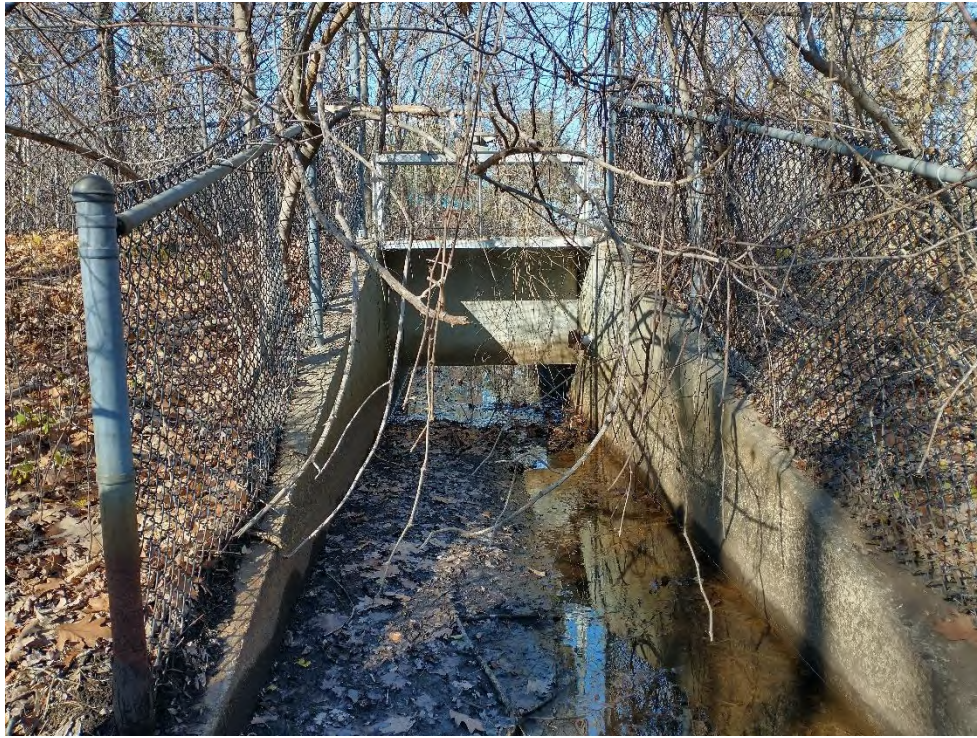
Figure 4: Concrete sluiceway with gate leading into SNUP Basin 1
