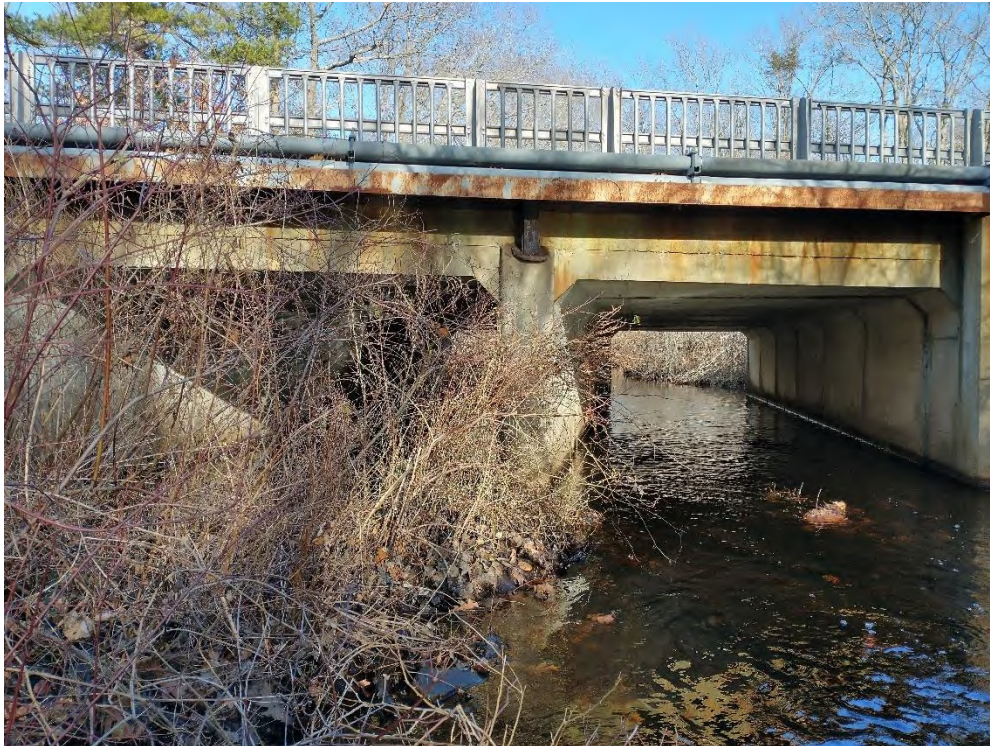
Figure 7: Upstream face of Libbey Industrial Parkway twin box culvert
