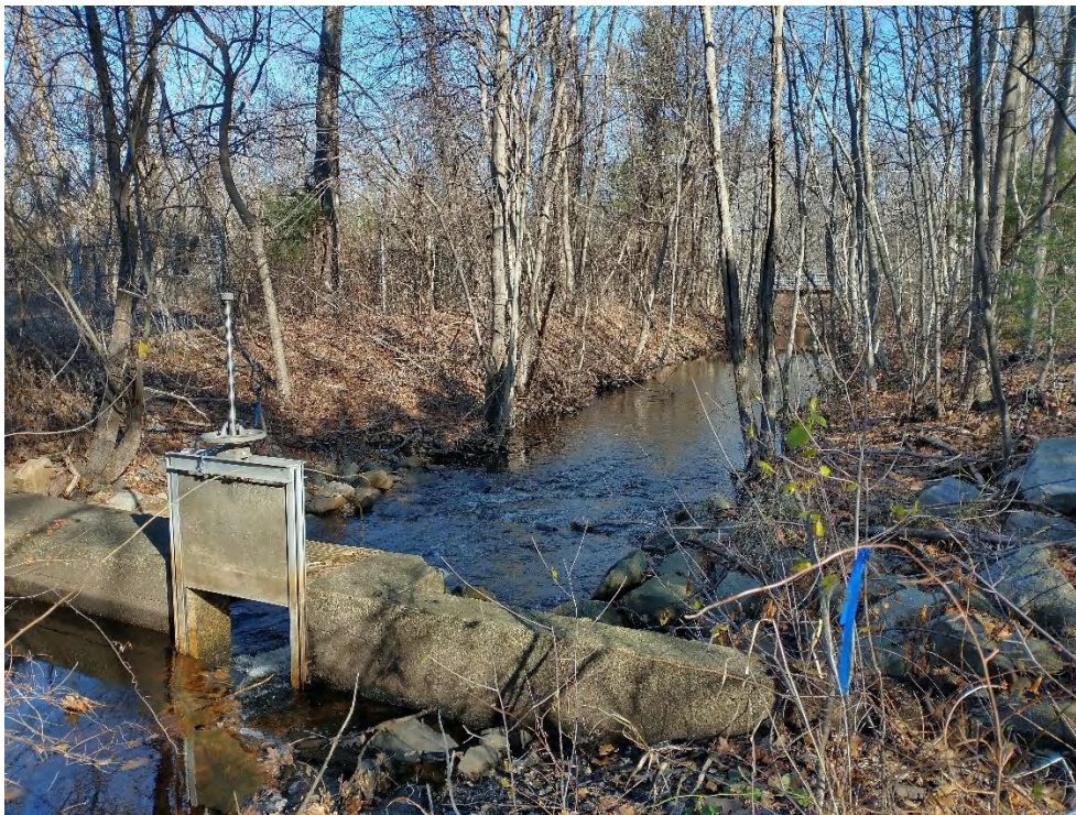
Figure 3: Existing concrete dam with metal gate
