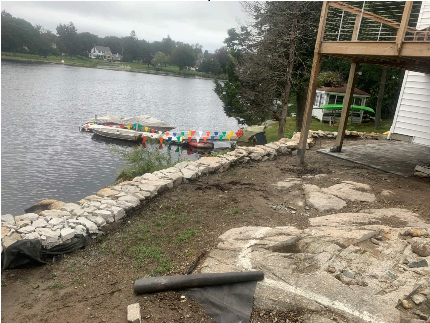
Photo 5: Rear yard area
