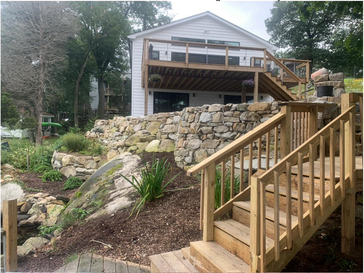
Photo 3: Home and Stone Retaining walls in rear yard
