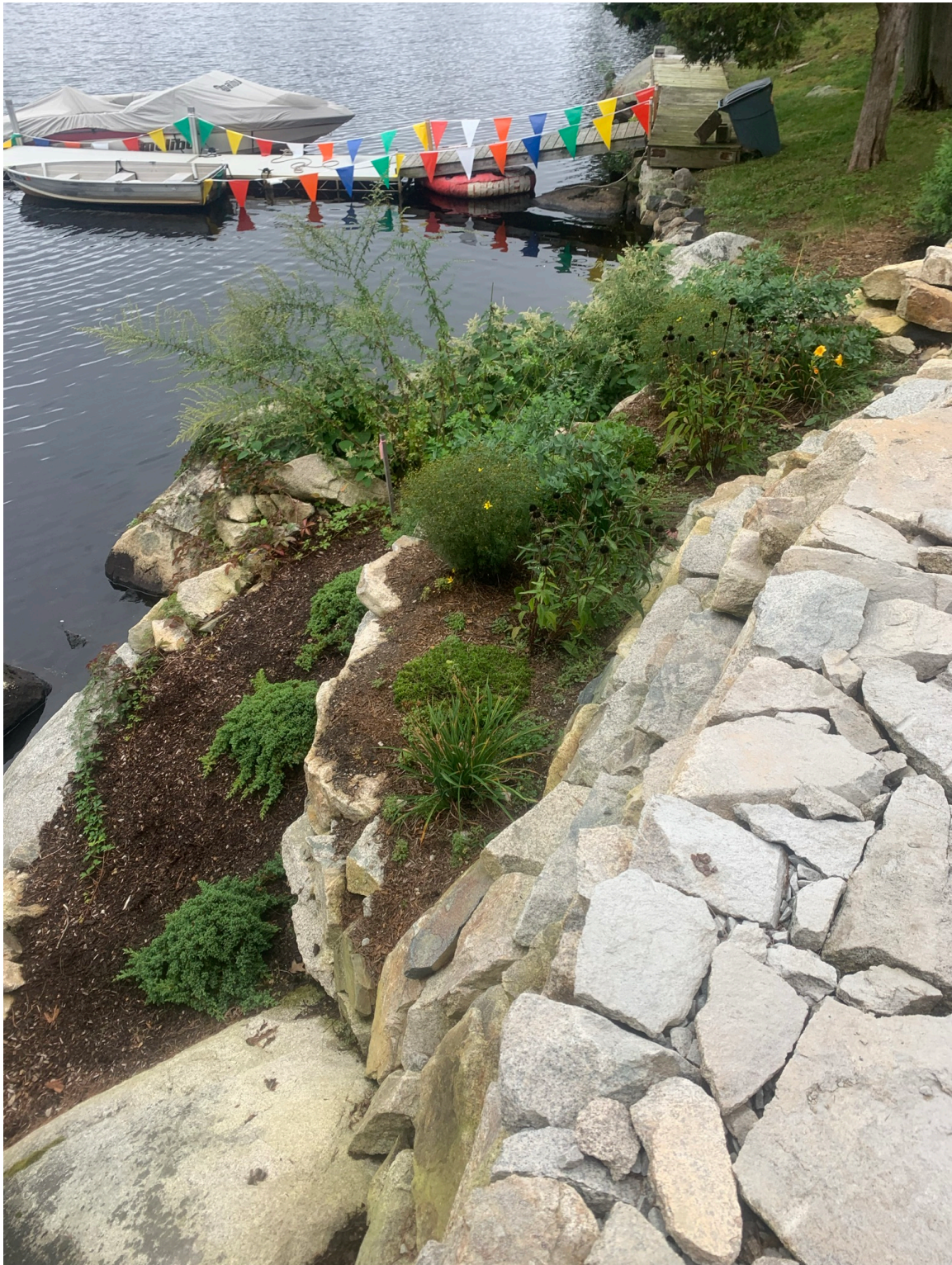
Photo 6: Rain Garden Area
