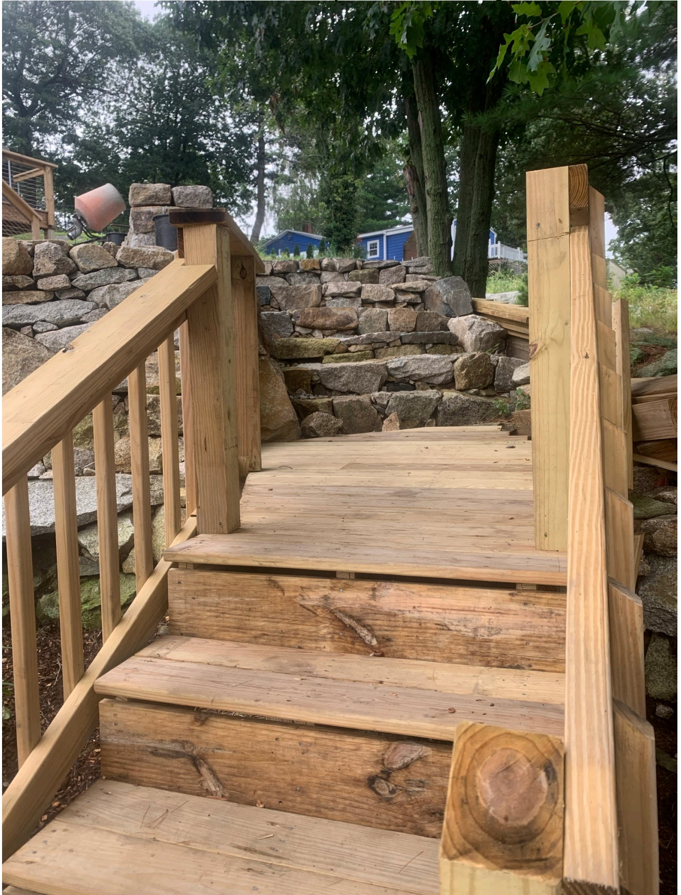
Photo 4: Stairs and walkway from home to existing deck
