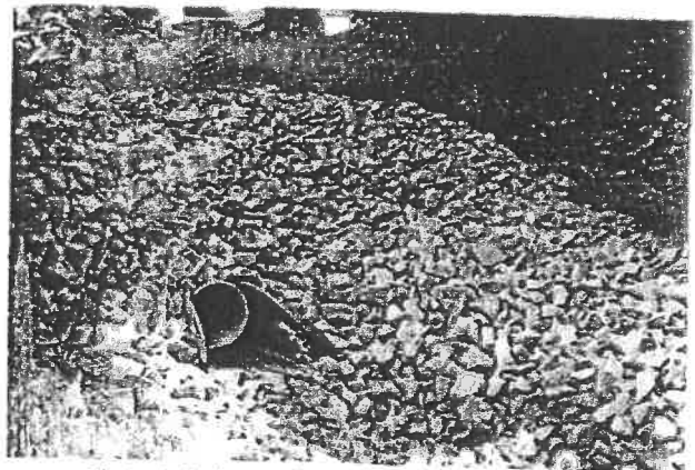
Photo 2: Drainage pipe on east embankment, looking west (Source: site visit June 2018)
