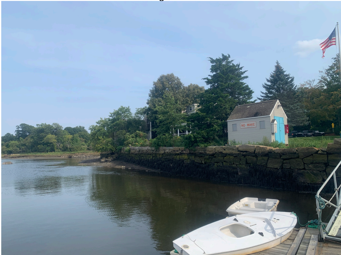
Photo 6: Retaining wall and tidal flat area
