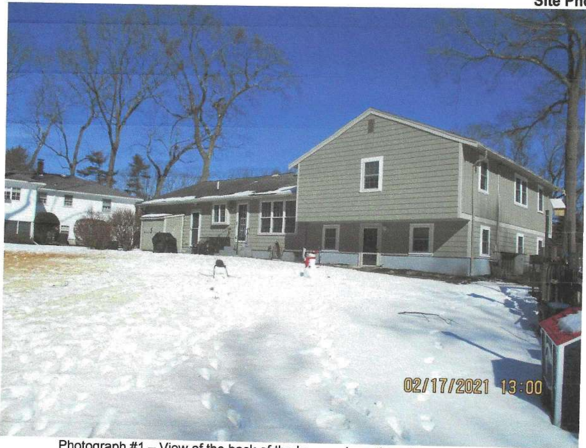
Photograph #1 – View of the back of the house where the addition is proposed.
