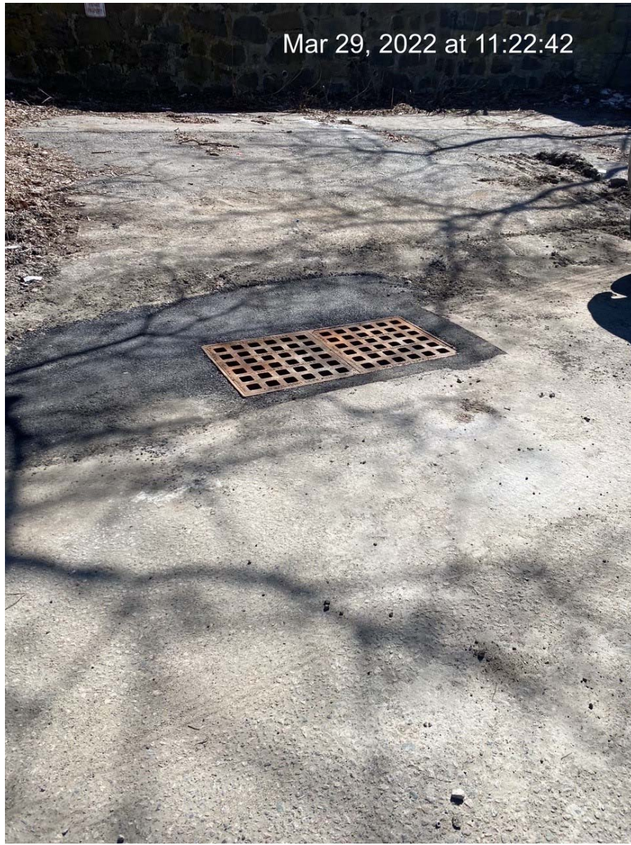
Photo 1 – Installed Off-Site Double Catch Basin
