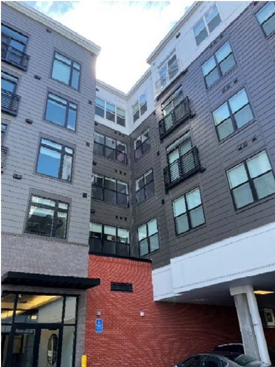
View of building intersection facing True North.
