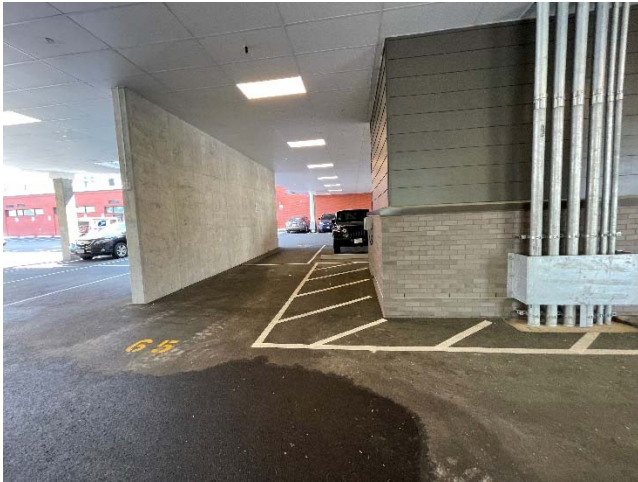
View of parking lot under building facing East.
