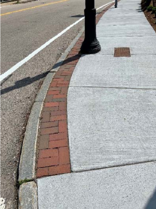
Sidewalk flush to curb facing West.
