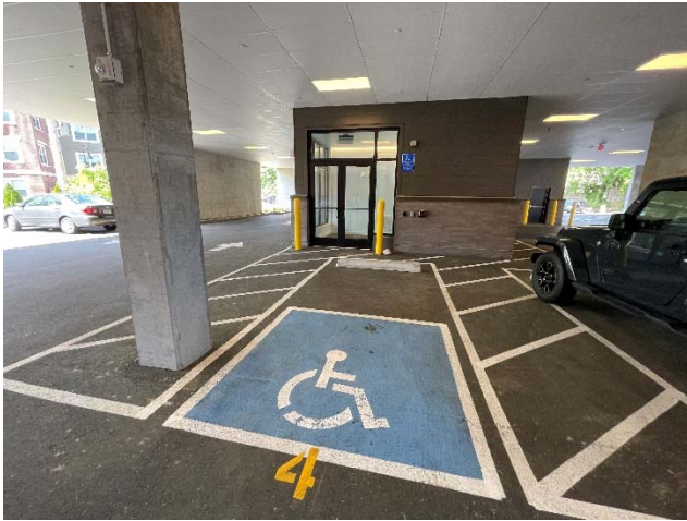
View of parking lot from opposite side of Location 7 facing West. Building entrance and handicapped parking in view.
