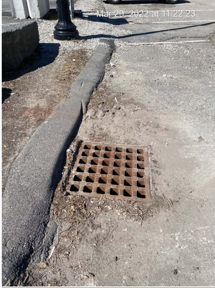
Photo 4 – Existing Off-Site Catch Basin
