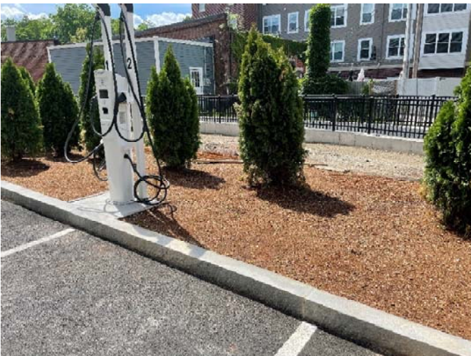
View of curbing, planted trees, and car charging station facing West.
