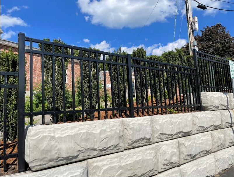
View of top of retaining wall and fence. Facing south-southwest.
