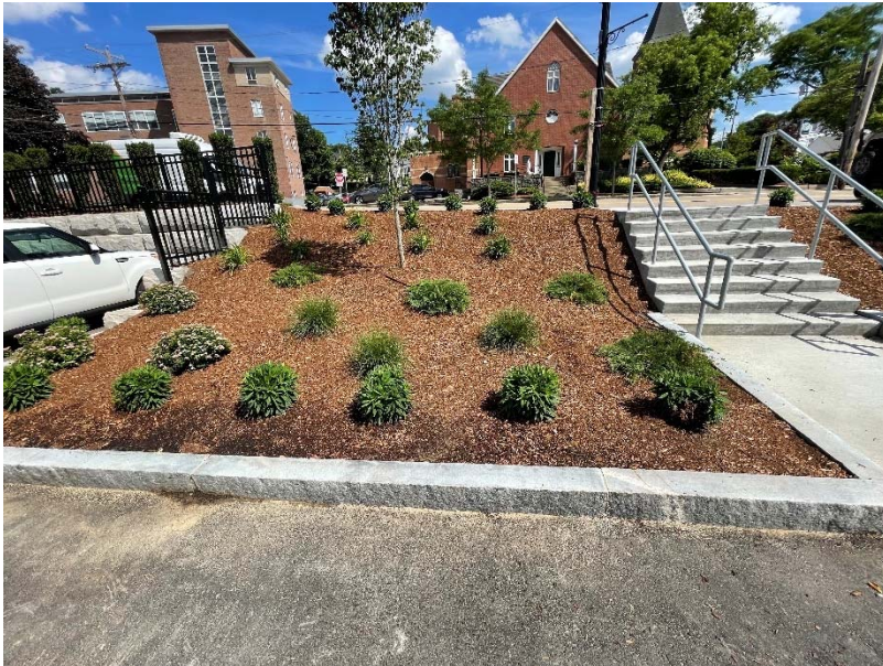
View of Landscaped area and stairs with guardrails facing Southeast.
