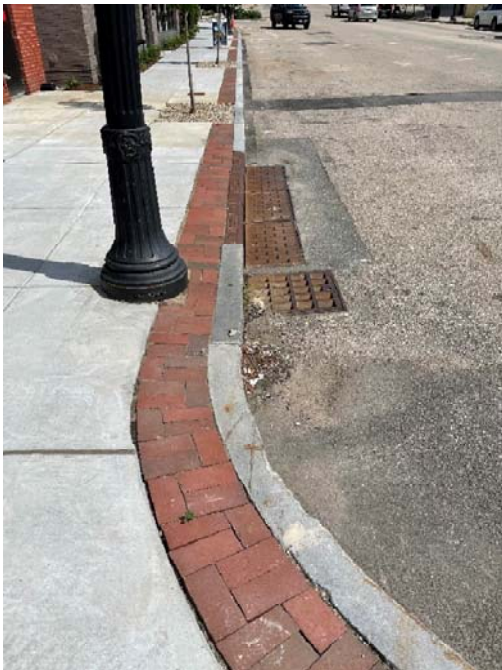
Curb and sidewalk view.
