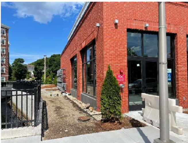
View of side of building looking North-Northeast from Washington street.
