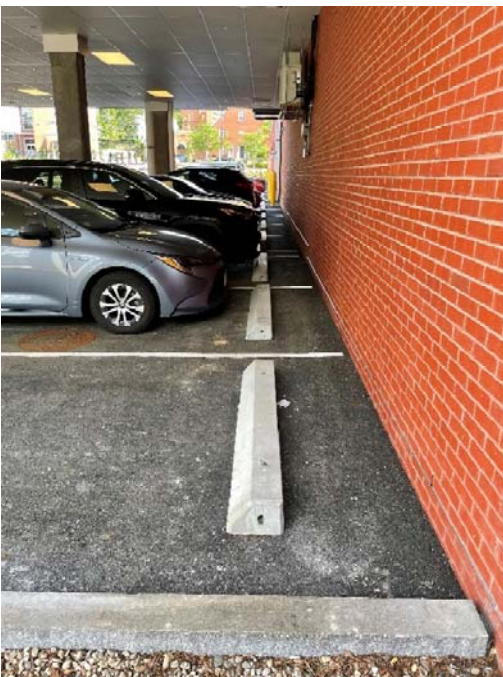
View of parking curb stops under building facing east.
