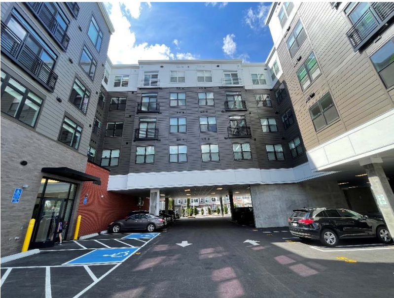
Facing Northwest, view of drive aisle under building, building face, bollards, and support structures.
