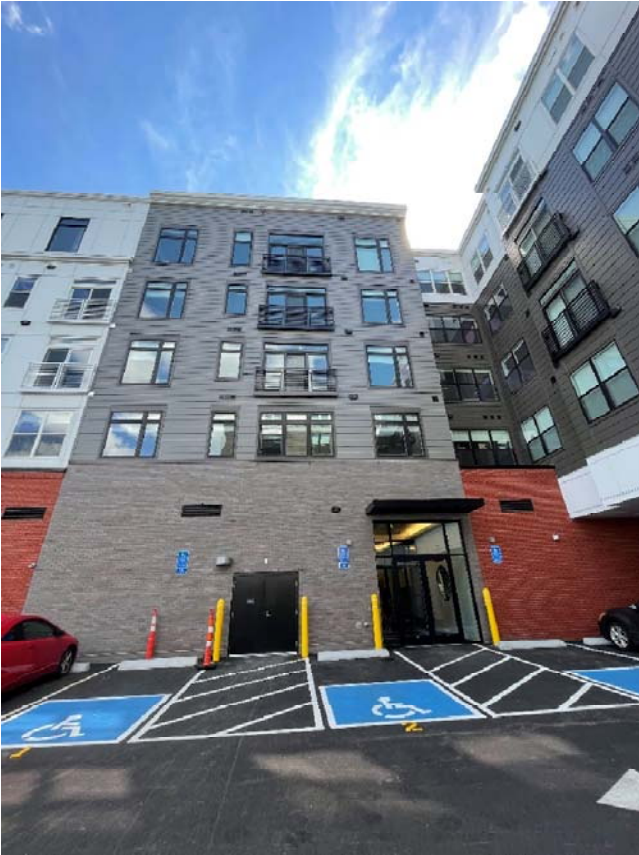
Facing West, slightly Northwest, view of building face and building intersection.
