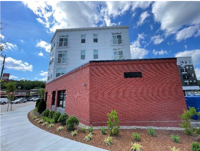
View of building and landscaped bed and plantings on Commercial Street facing Northwest.
