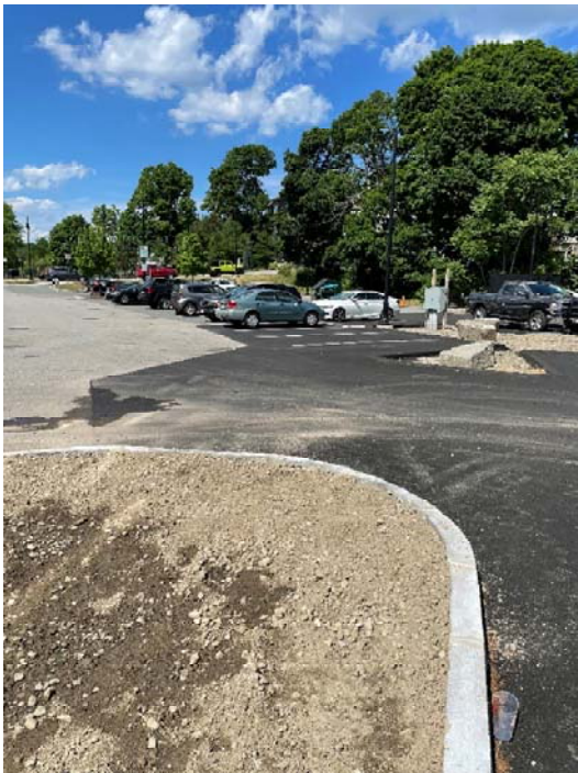
View of freshly paved pavement meeting existing pavement. Facing South-Southwest.
