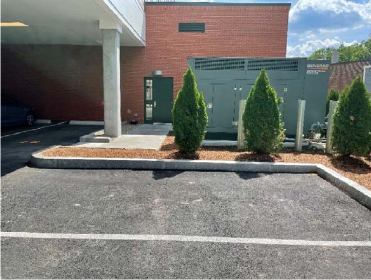
View of building entrance, curb, planted trees, and building support column.
