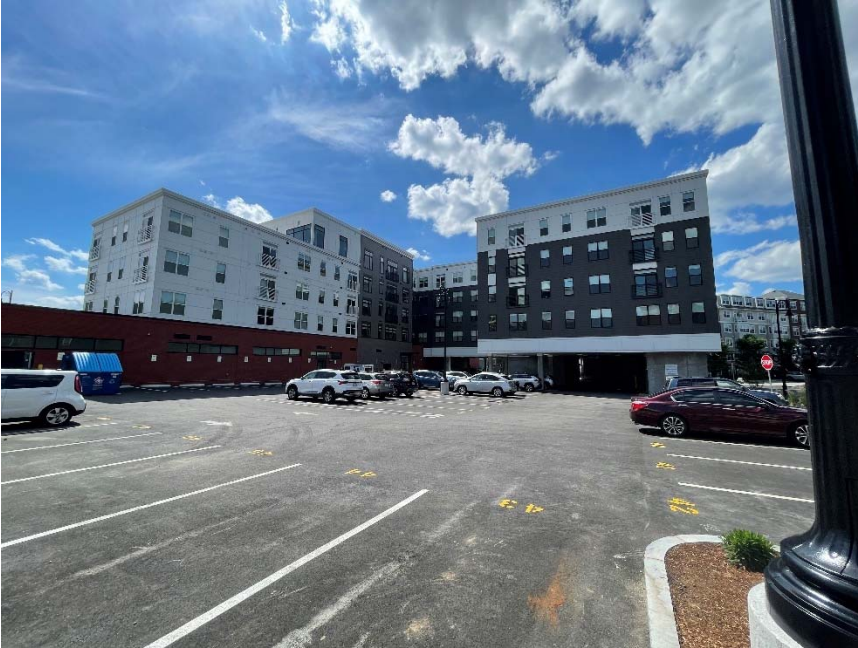
View of building and parking lot facing North-Northwest.
