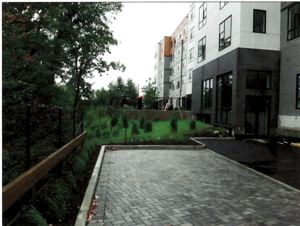
VIEW OF LOOKING SOUTH OF SOUTHEAST CORNER OF POROUS PAVER PARKING AREA TOWARD POOL AND AMENITIES AREA
