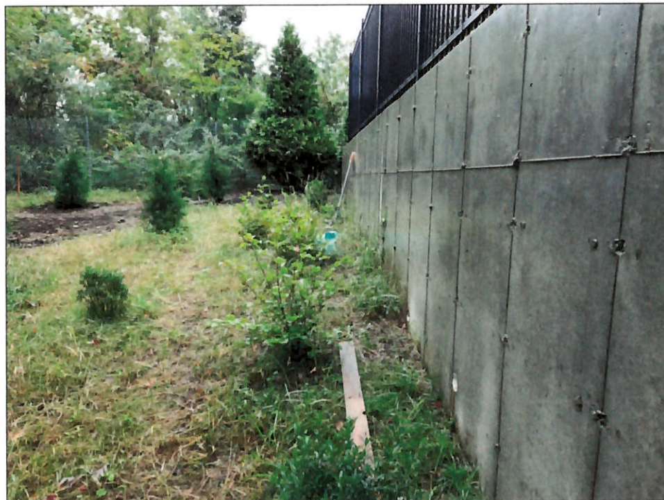
VIEW OF LOOKING SOUTH OF RETAINING WALL AND AREA BEHIND POOL
