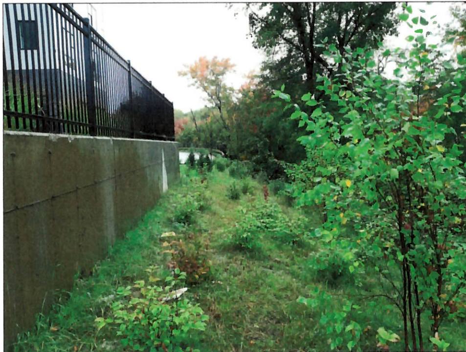
VIEW OF LOOKING NORTH OF AREA BEHIND AMENITIES AREA
