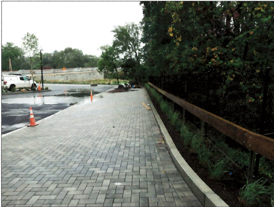
VIEW LOOKING NORTH OF POROUS PAVER PARKING AREA AT NORTHEAST CORNER OF SITE
