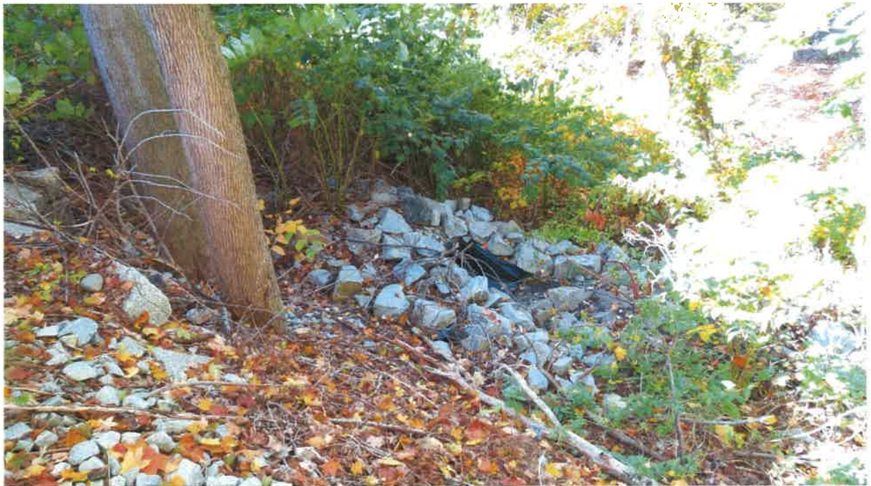
Looking Northwesterly from Slope to Stormwater Outlet and Stilling Basin
