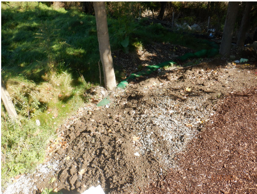
Photograph 8: Area of bare soil at northeast corner of property.
