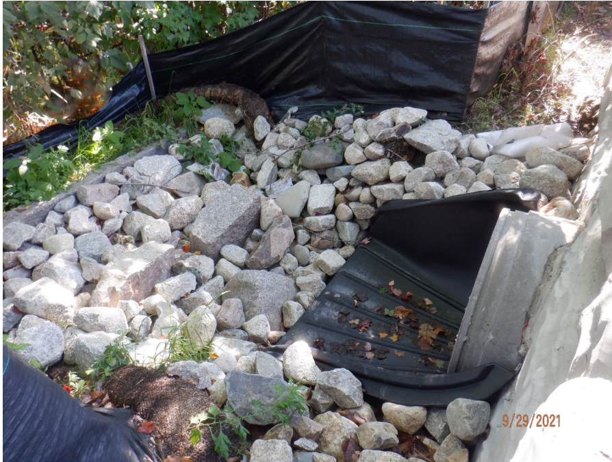
Photograph 11: Stormwater outlet #1 and erosion control barrier.
