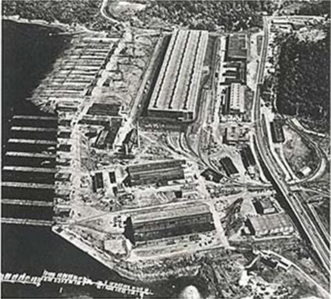
Figure 6-11. Hingham Shipyard, Weymouth Back River 1940s. View is looking toward the east with the mouth of the Back River toward the top of the figure. Source: Hingham Historical Society.
