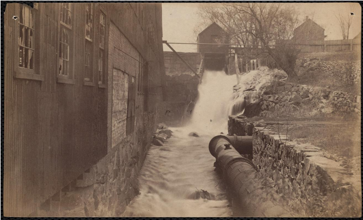
Figure 5-5. Upper Falls of Weymouth Iron Works. The house at the top center of the picture encloses a water wheel for capturing energy from the flow of water out of Whitman's Pond. Modified from digital image from Weymouth Public Libraries Historical Photograph Collection (Digital Commonwealth, Massachusetts Collections Online, accessed March 11, 2016).
