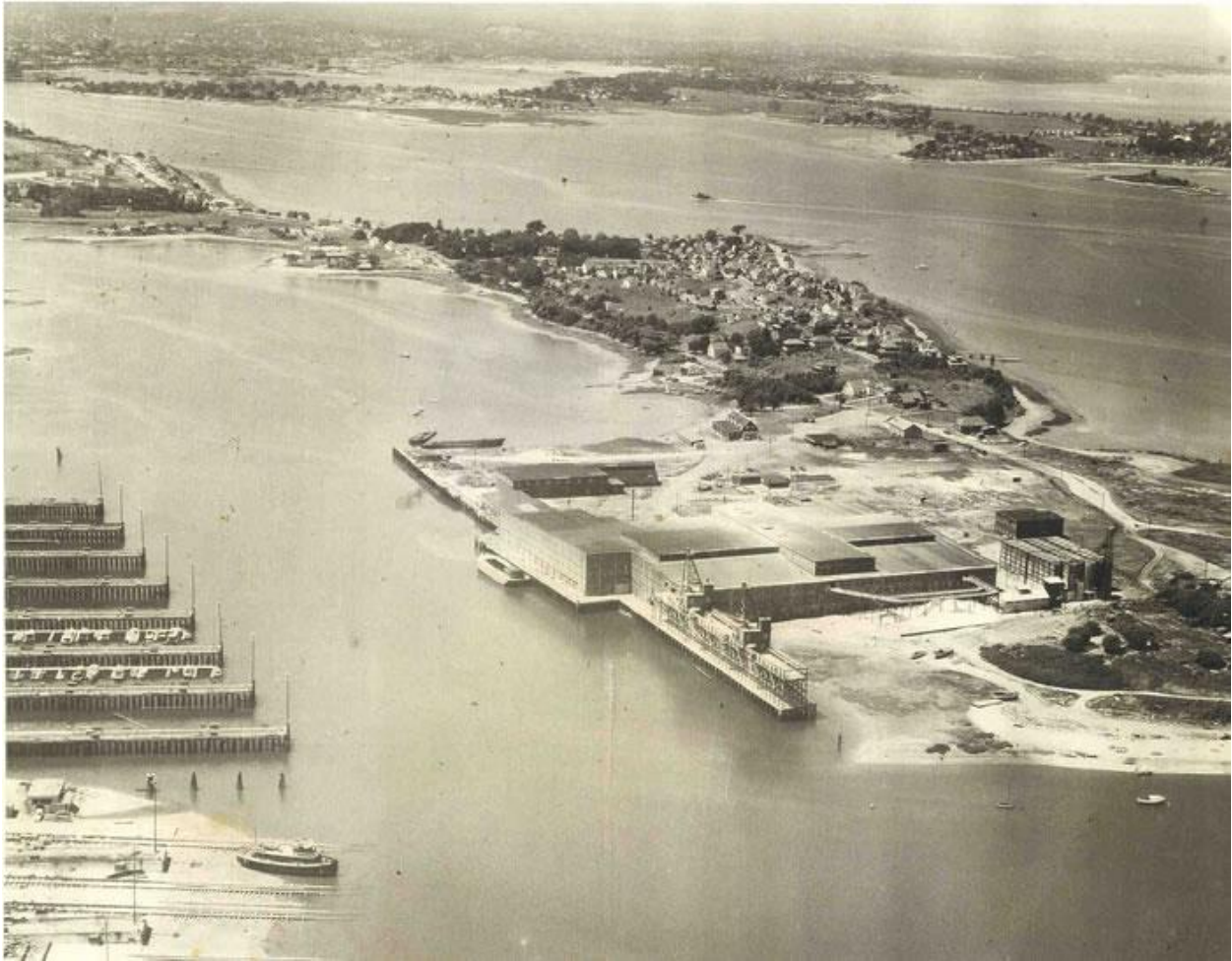
Figure 6-6. Bradley/Agrico Fertilizer Plant, Weymouth Neck. Fertilizer plant is shown in the center of the picture; view is looking south along Weymouth Neck. The docks of the Hingham Shipyard can be seen on the opposite shore (left side of picture). The current Webb Memorial Park would be located just off the right side of the picture. Source: Weymouth Historical Society.
