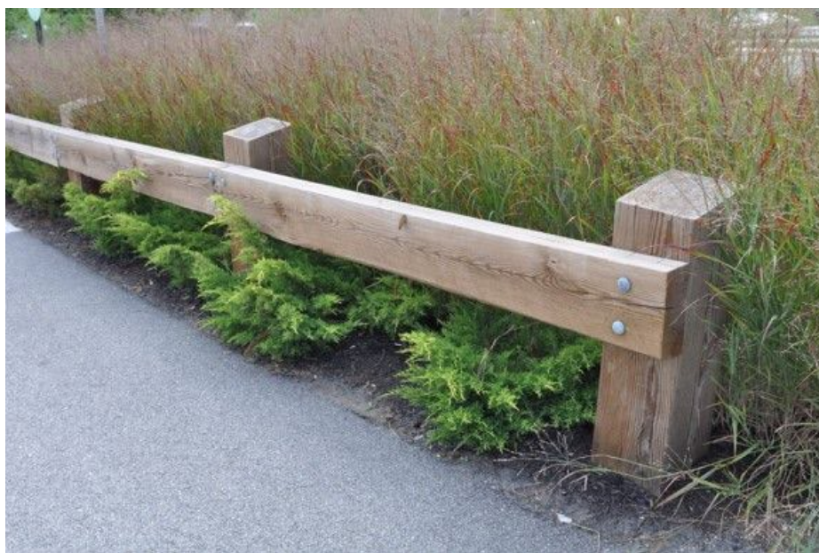
Figure 7-4.1: Trail Perimeter Guardrail
