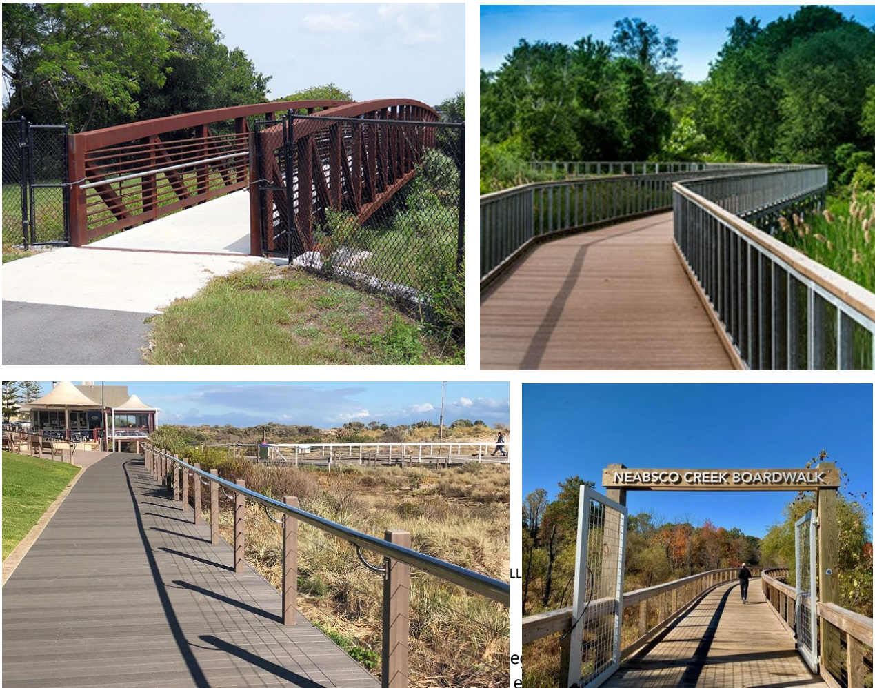
Figure 7-7: Boardwalk Trail Railing
