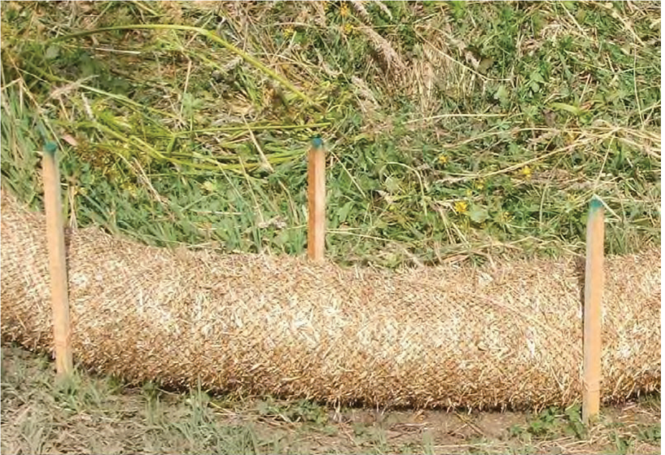
STRAW WATTLE – SHALLOW SLOPE ( \leq 4:1 ) (ALTERNATE STAKING)
