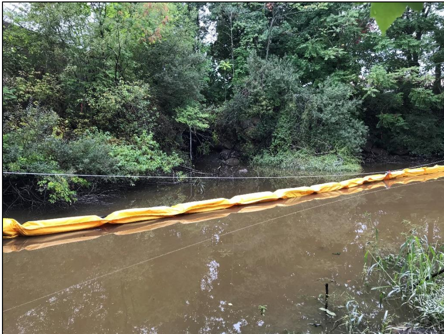
Photo 5. Culvert outlet, showing work area prior to construction 9/13/2022
