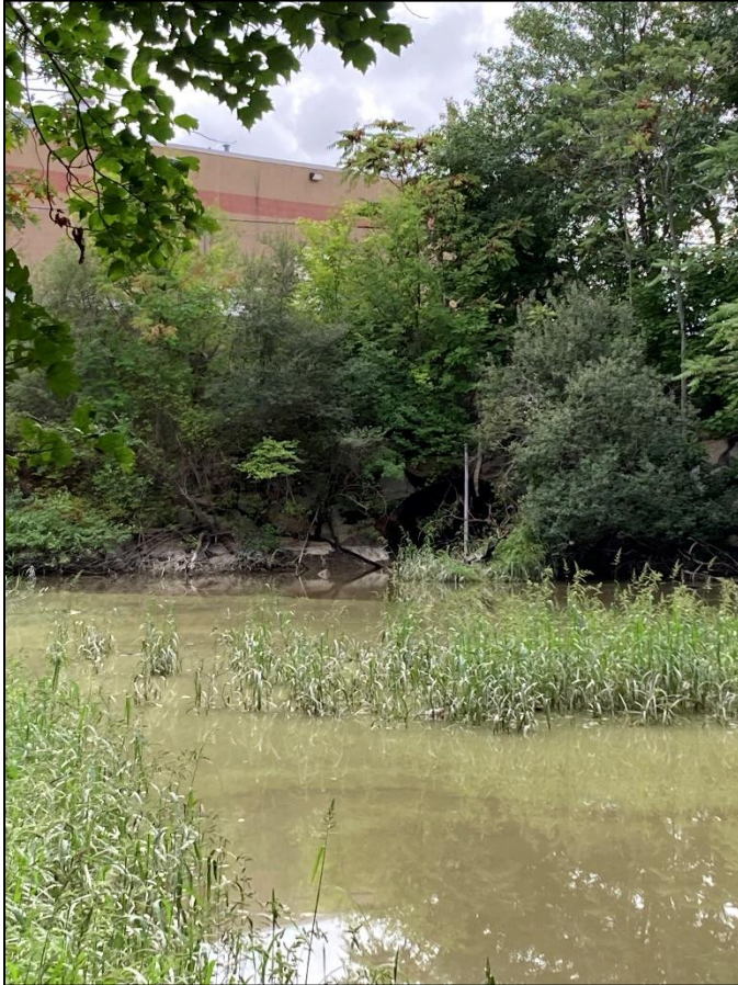
Photo 3. View toward culvert outlet 9/7/2022
