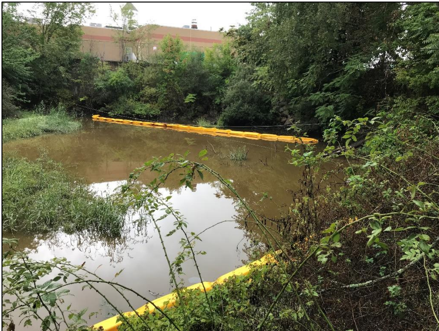
Photo 4. View toward culvert outlet, with turbidity curtains installed 9/13/2022
