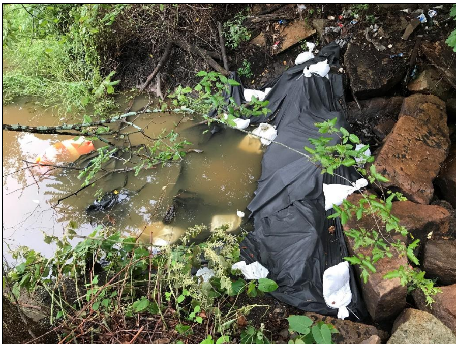
Photo 6. Rock dam at downstream side of impoundment 9/13/2022
