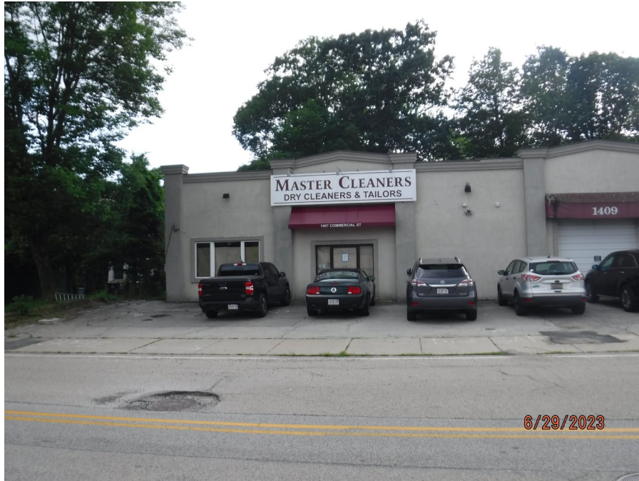
Photograph 21: View of Site D, facing the existing building, along Commercial Street.
