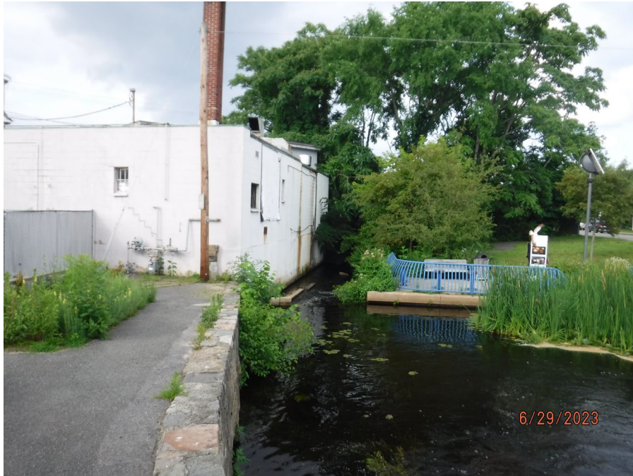
Photograph 19: View of the east side of Site C, along the Herring Run Pool Park, facing north.
