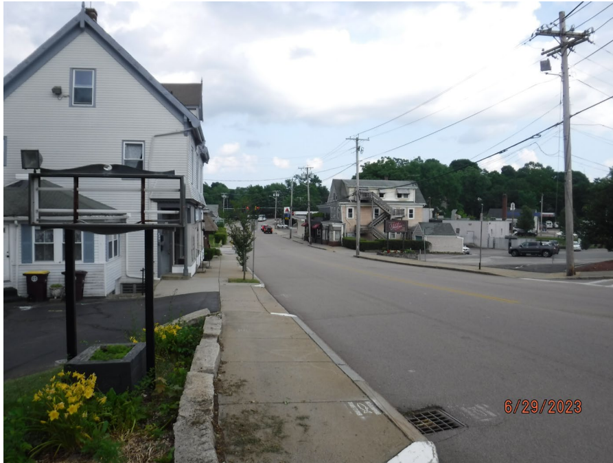
Photograph 11: View of the front of Site A, along Broad Street, facing east.
