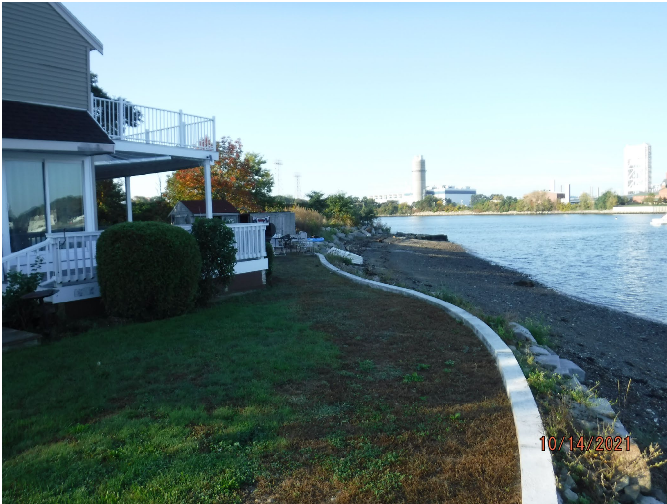
Photograph 2: View of the concrete fence foundation and lawn, facing south.
