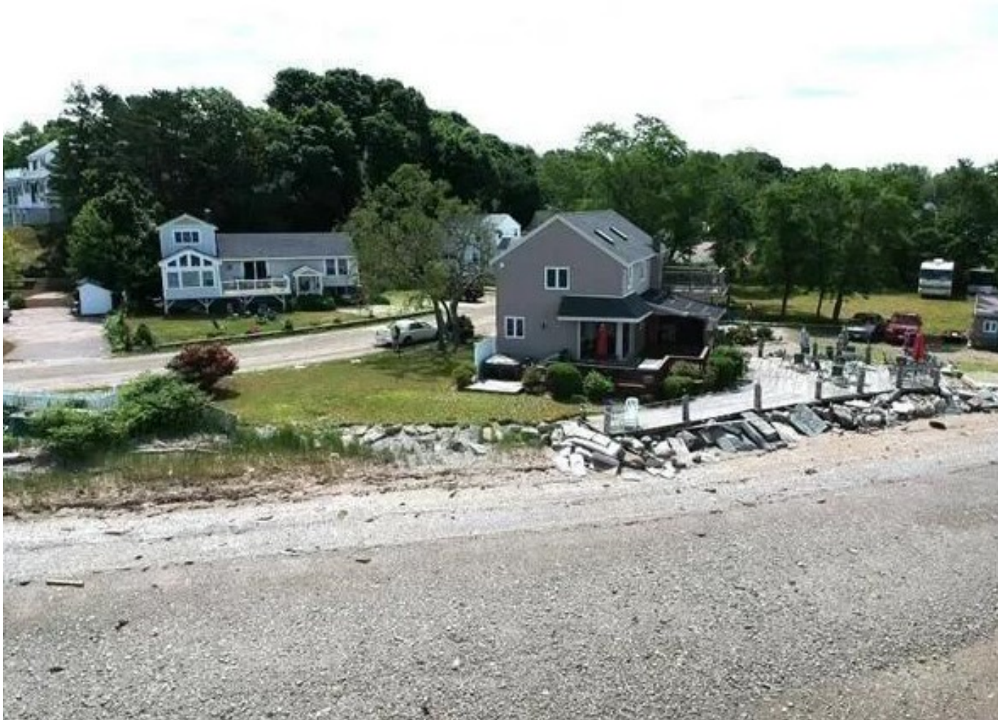
Photograph 5: View of the resource areas prior to construction of fence foundation. Note pre-existing structure (deck) along Coastal Bank.
