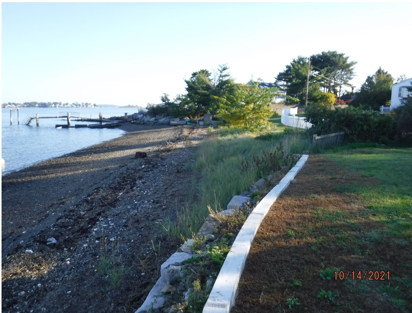
Photograph 3: View of the concrete fence foundation, Coastal Beach, Coastal Dune, and lawn, facing northeast.
