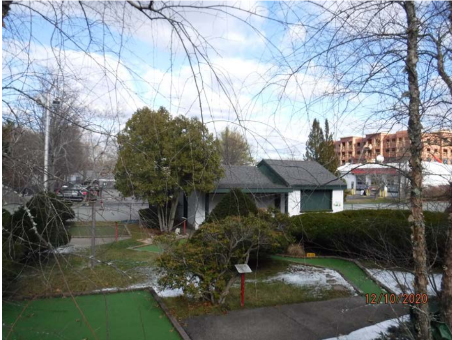
Photograph 1: Overview of existing conditions within the miniature golf course looking north.
