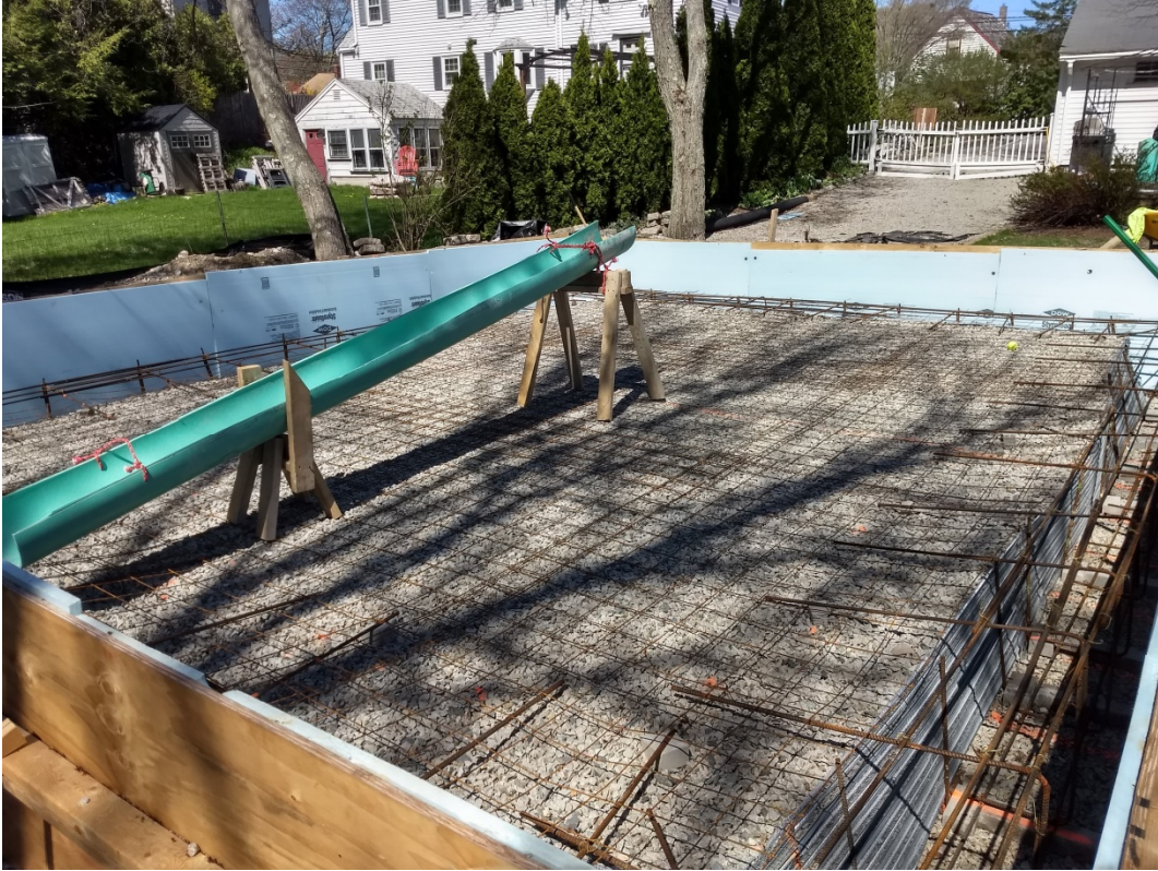
Stone Subgrade Prior to Concrete Slab Placement
