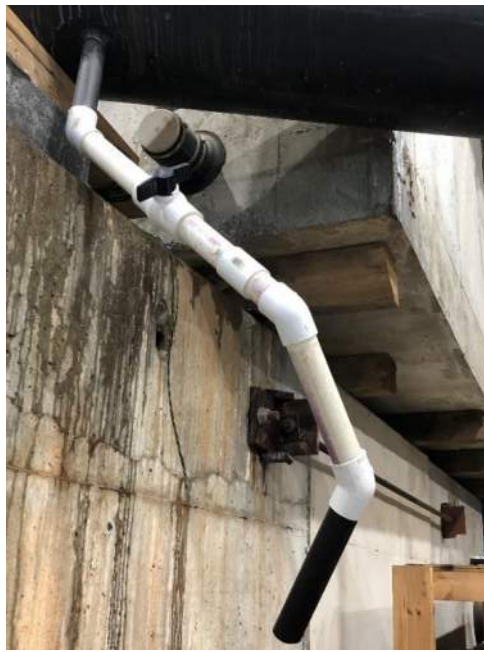
Figure 8 Photograph of Background Sampling Port
