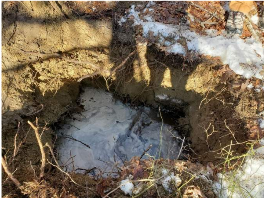
Photo 11: View of Test Pit SH-TP-19.
