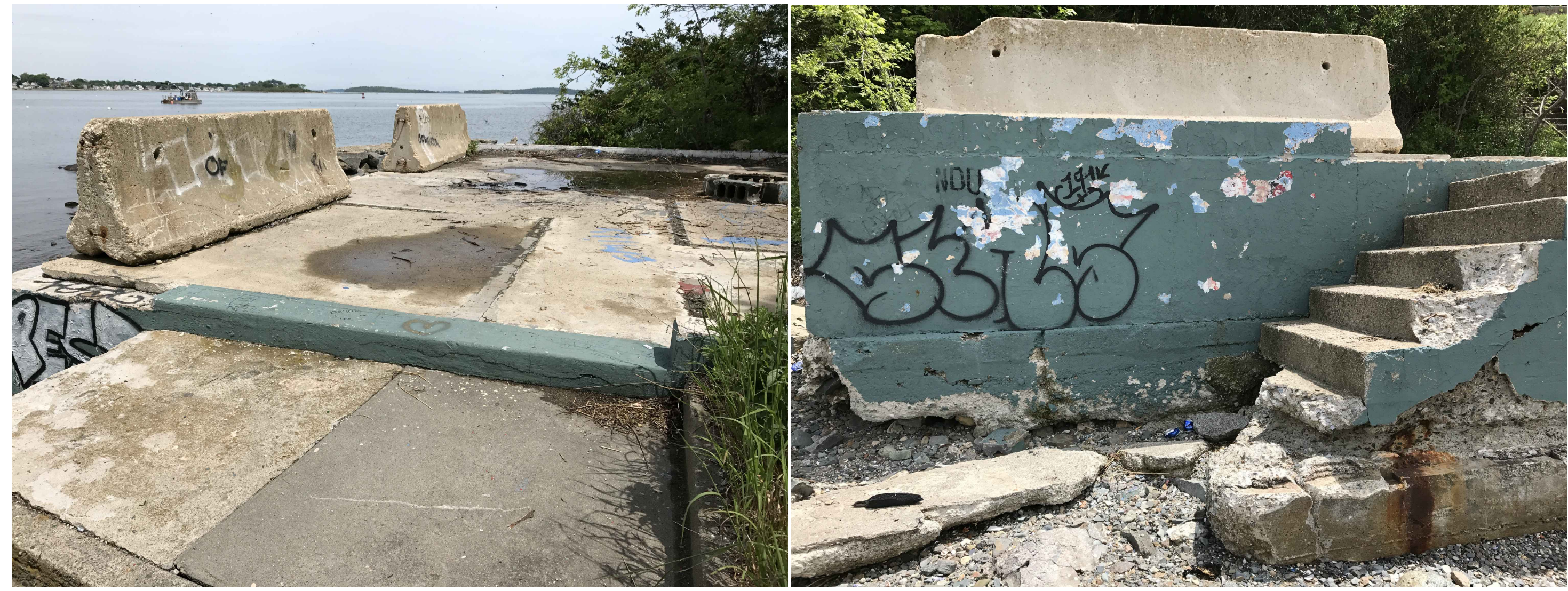
PHOTOS NEAR SECTION B-B
