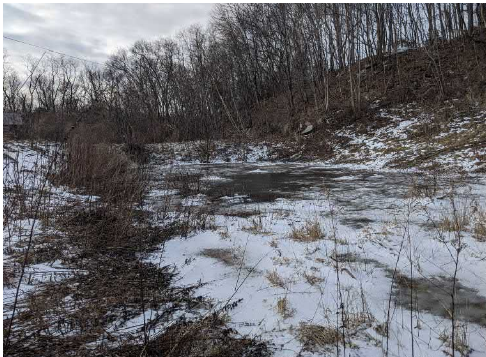
View of the stormwater basin to the northeast of the incinerator—facing south.
