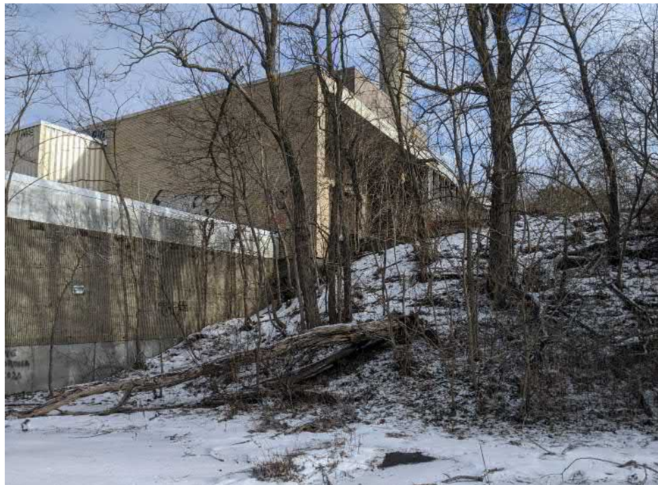
View of the incinerator from the south—facing north.
