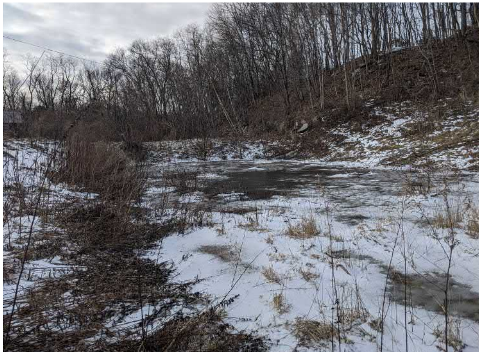
View of the stormwater basin to the northeast of the incinerator—facing south.
