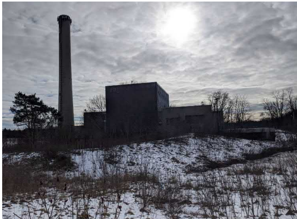
View of the incinerator and adjacent stack—facing southeast.
