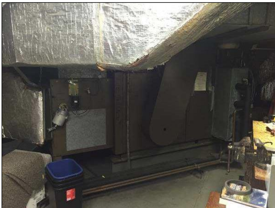
Figure 35: Indoor air handling units (more than 50 years old).
