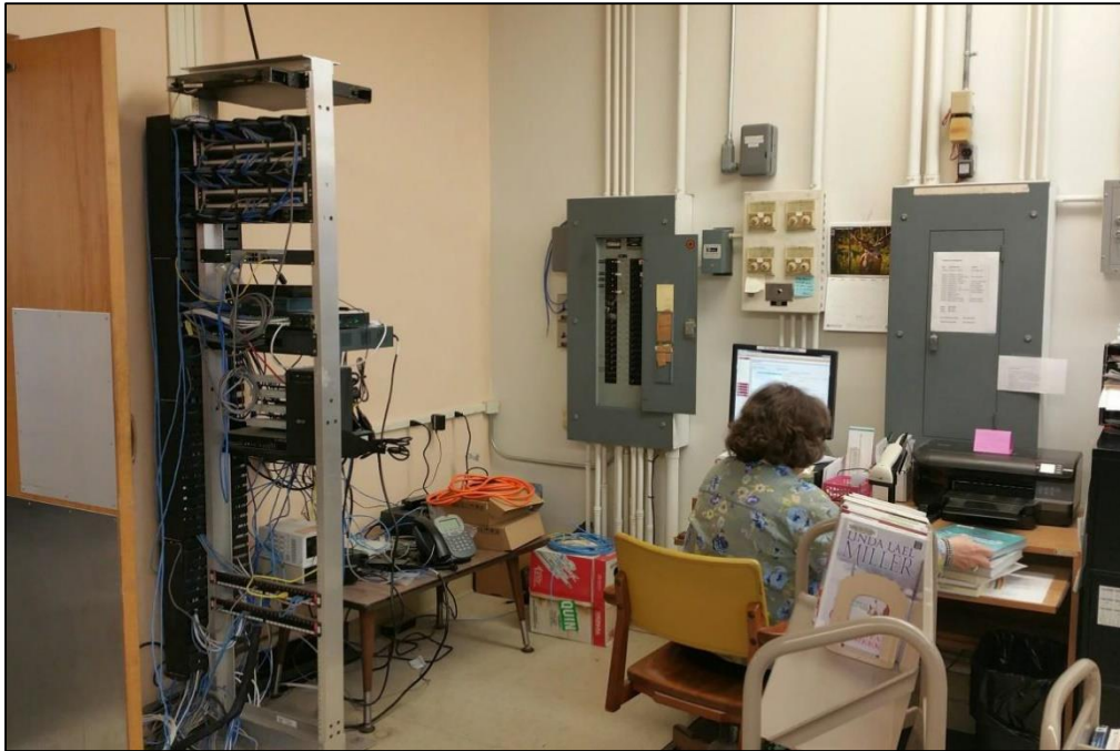
Figure 26: Staff desk situated next to data servers and fuse boxes due to limited power and data outlets.
