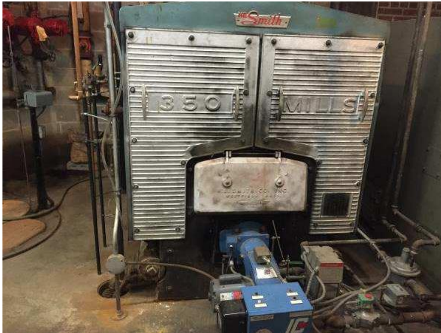
Figure 34: Gas-fired, cast-iron boiler (more than 25 years old).
