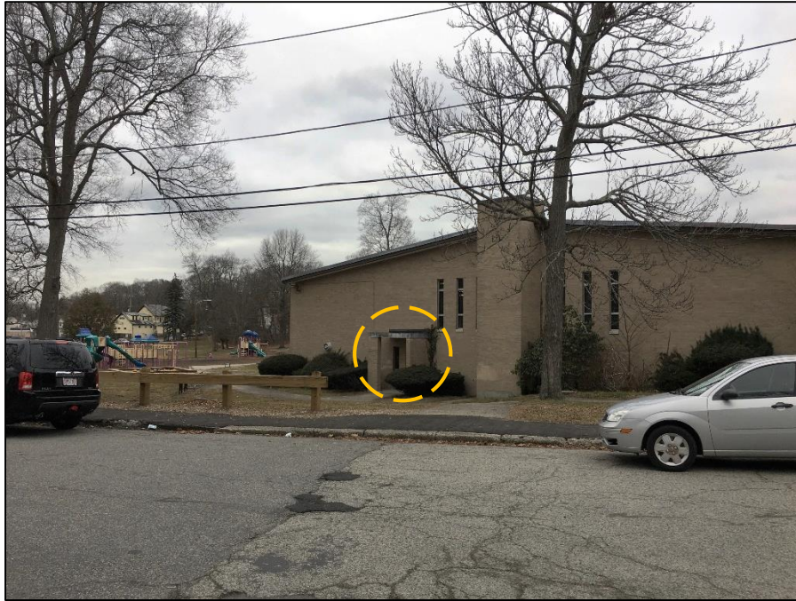
Figure 31: Side entrance facing west towards Franklin Street. Curb has no ramp, and pathway to entrance slopes down (not ADA accessible).
