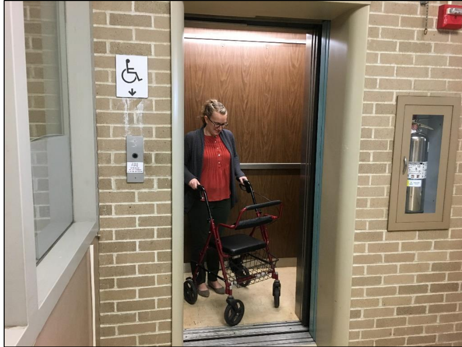
Figure 30: Elevator is very small and does not meet ADA guidelines.
