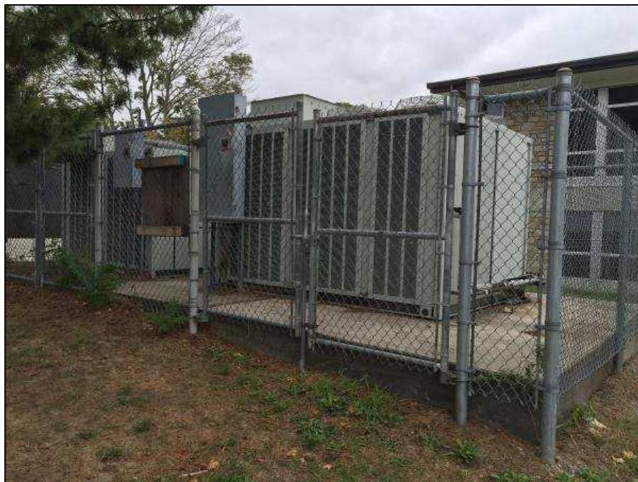
Figure 36: Outdoor, ground-mounted condensing units (approx. 28 years old).
