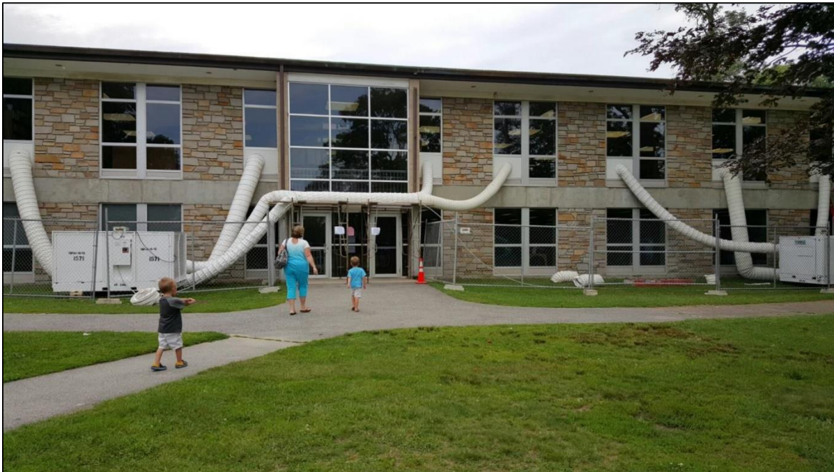
Figure 20: Back entrance facing Weston Park with interim HVAC system during summer of 2015.
